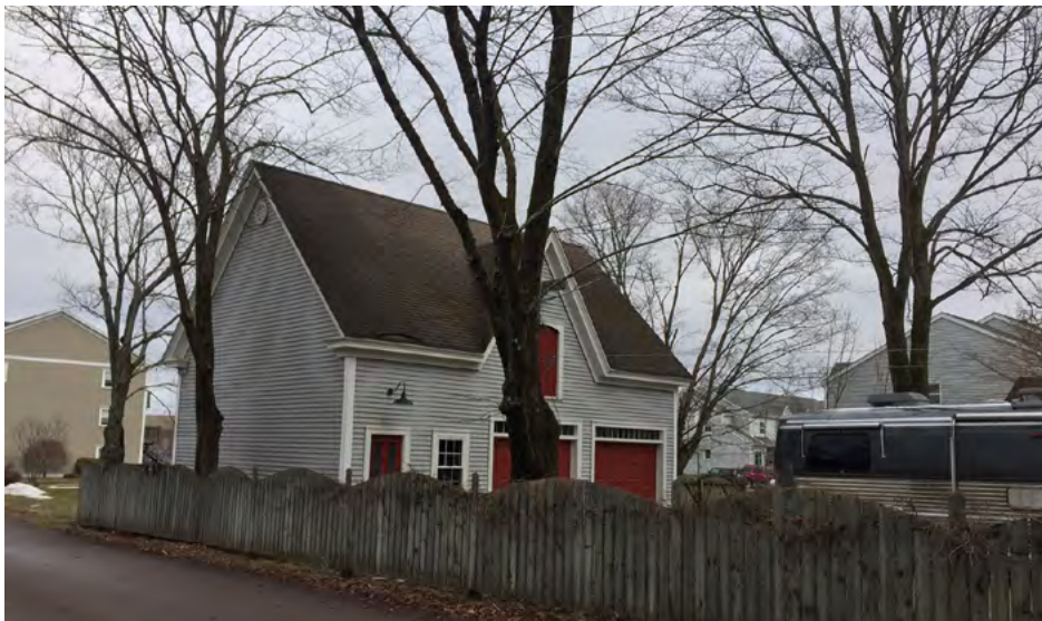
Photo of the Carriage House that is to be expanded as part of this development application. Taken from the driveway of 59 Queen Street.
