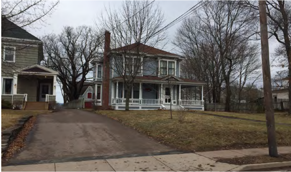
Photo of the subject property looking northeast from Queen Street
