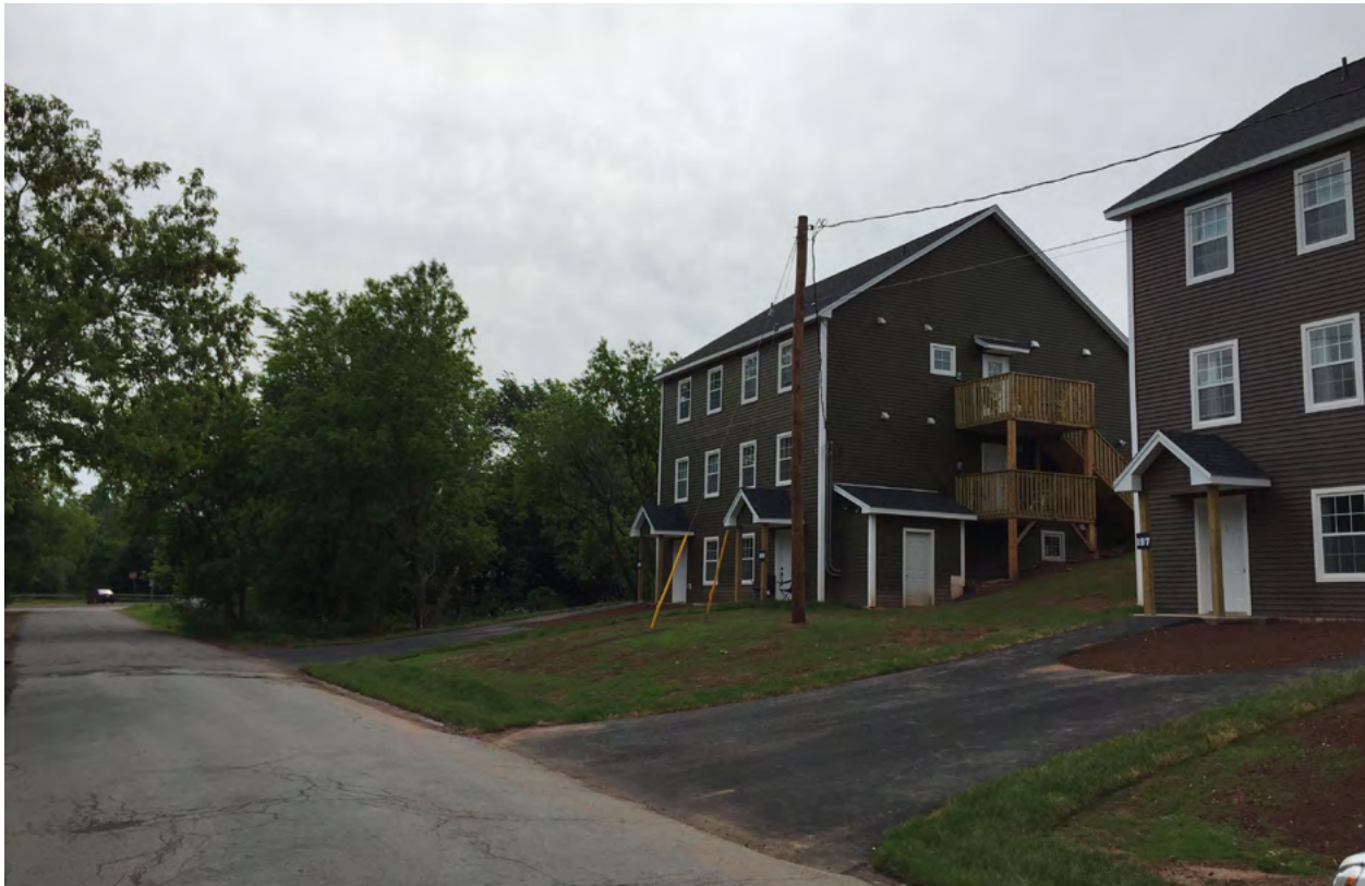
Photo of the subject property looking east from the former DAR right-of-way showing the two new 6-unit buildings on the subject property. The treed area to the left is the location of the proposed new 6-unit building.
