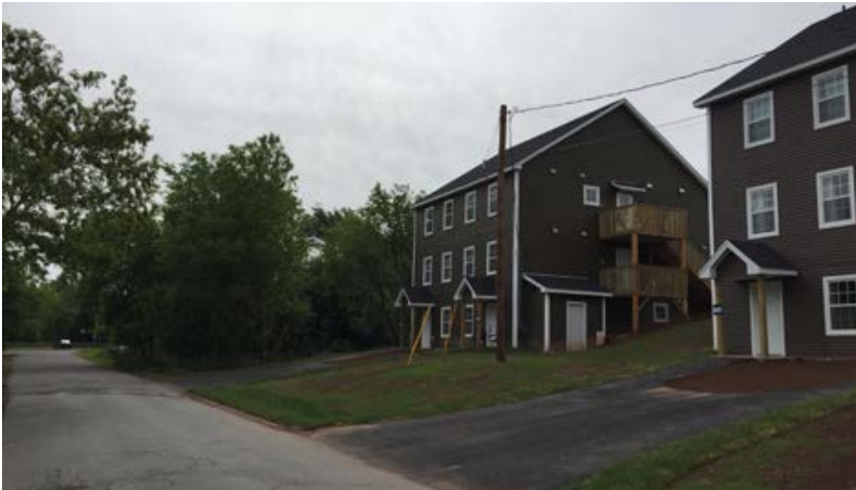
Photo of the subject property looking east from the former DAR right-of-way showing the two new 6-unit buildings on the subject property. The treed area to the left is the location of the proposed new 6-unit building.
