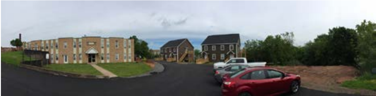
Panoramic Photograph of the subject property looking northwest towards Willow Street showing the 14 unit converted medical clinic to the left and the two existing 6-unit buildings at centre. The treed area to the right is the location of the proposed new 6-unit building.
