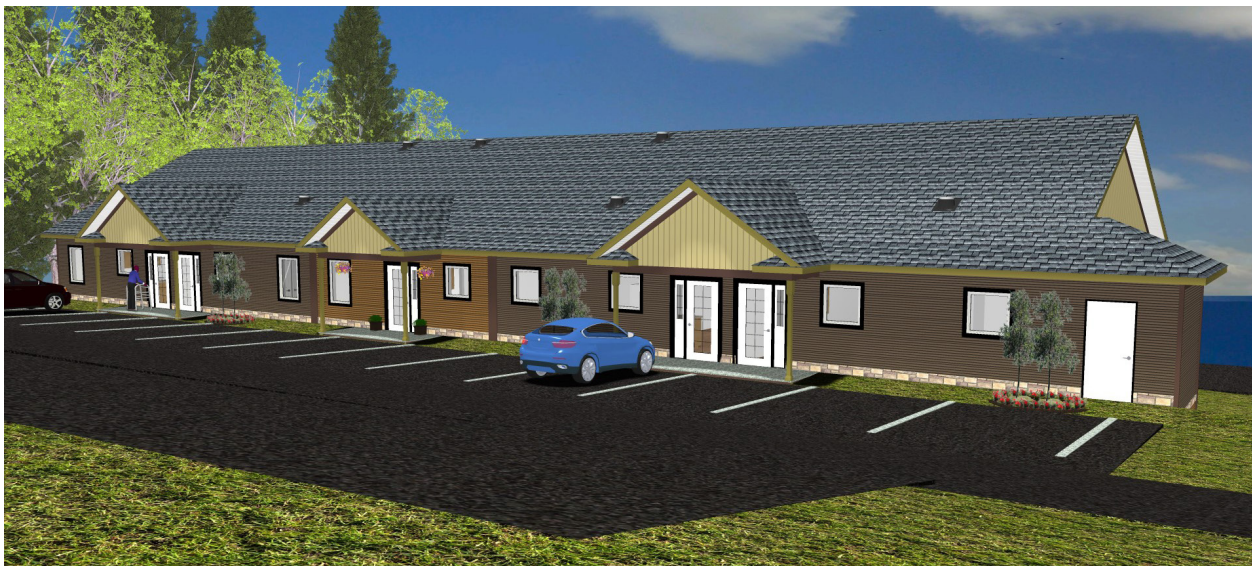
Rendering of the south, or uphill side of one of the six proposed 10-unit buildings. Due to the slope of the site, the structure is only one storey on this north side and the five upper level units are accessible at grade.
