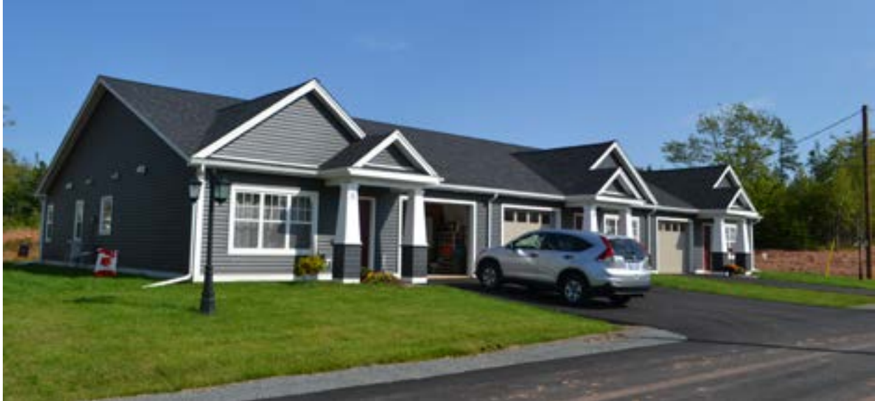
Photograph submitted by Meech Holdings Limited showing a three-unit one-storey townhouse style building. The four-unit structure proposed as part of the Philip Street development will use this same design and feature a similar exterior finish.
