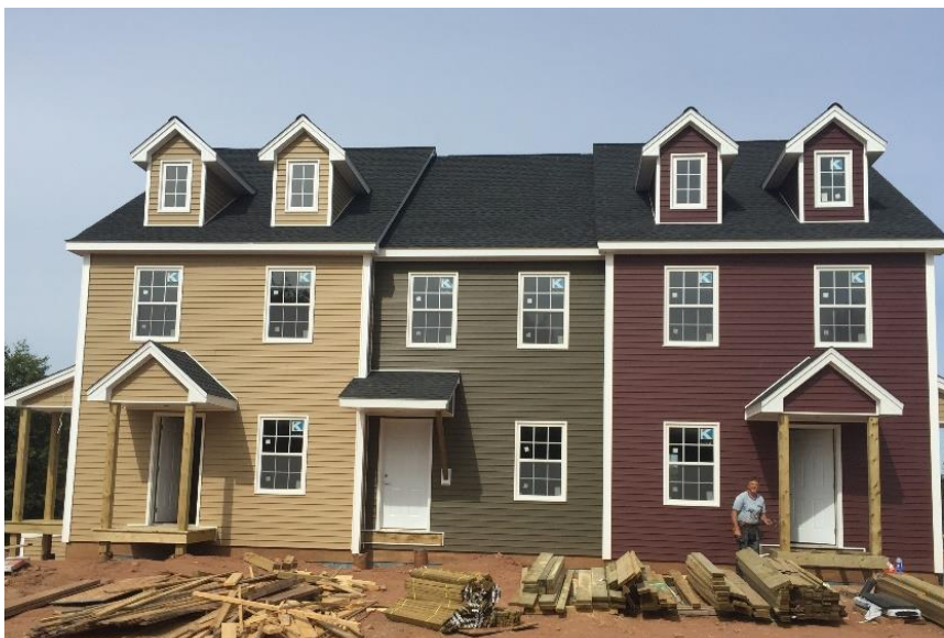
Two-Storey Three-Unit Dwelling
