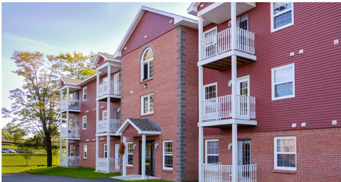
View of the three-storey main building facing Munroe Street
