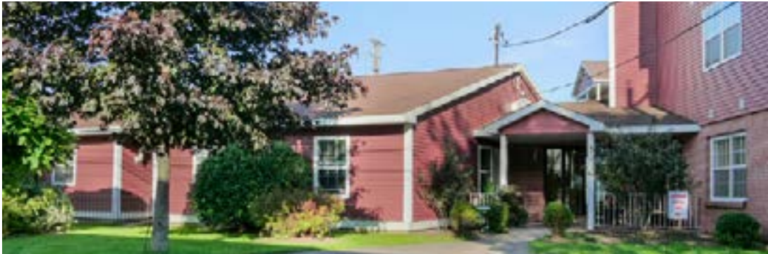
View of the one-storey building facing Munroe Court
