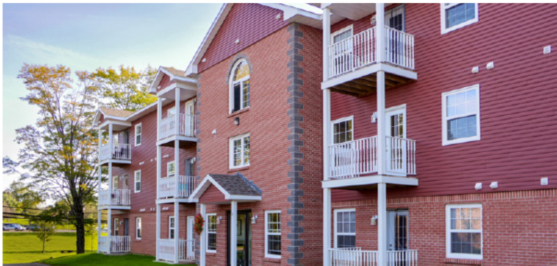
View of the three-storey main building facing Munroe Street
