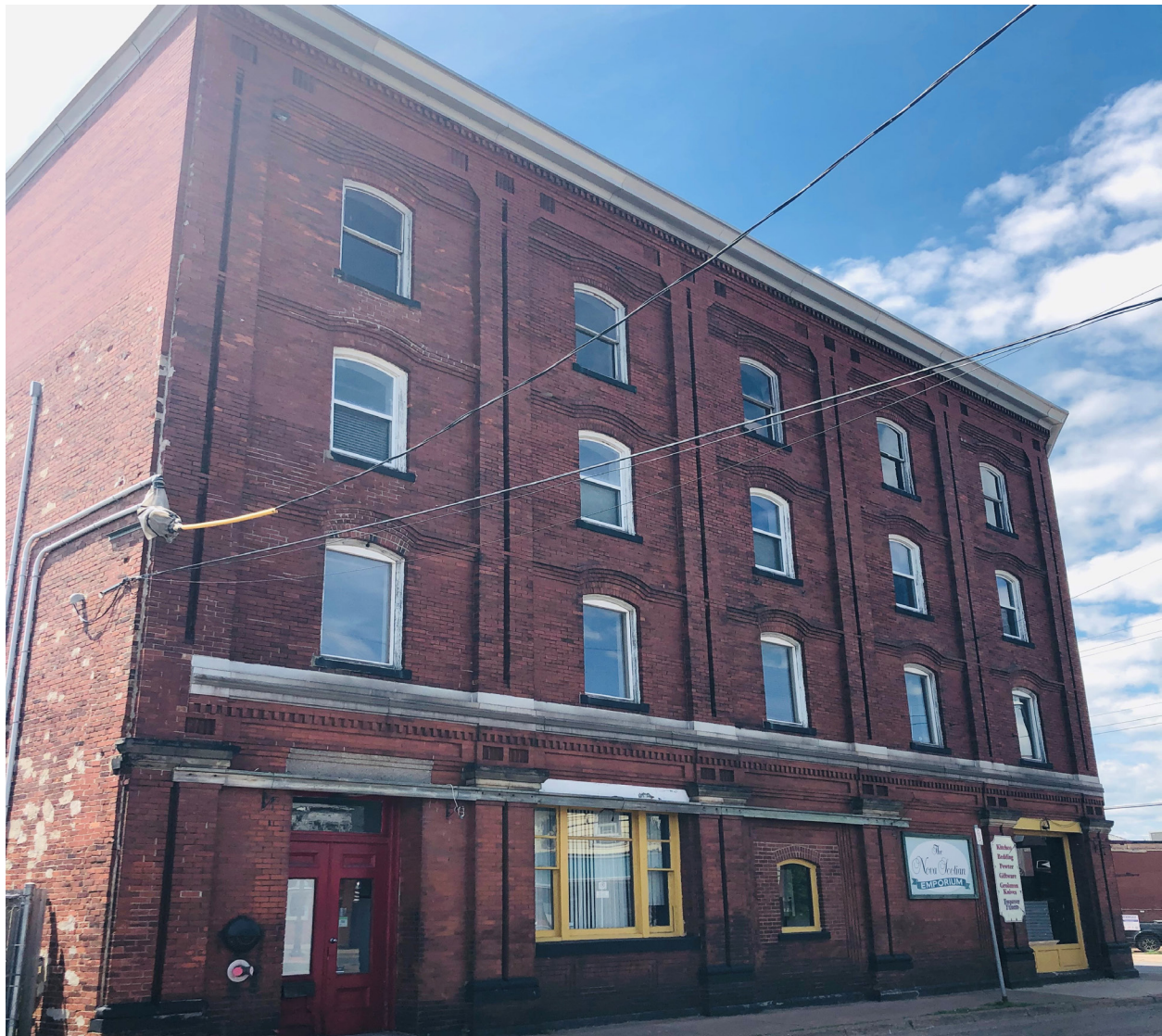
880 Prince Street looking northwest from Outram Street
