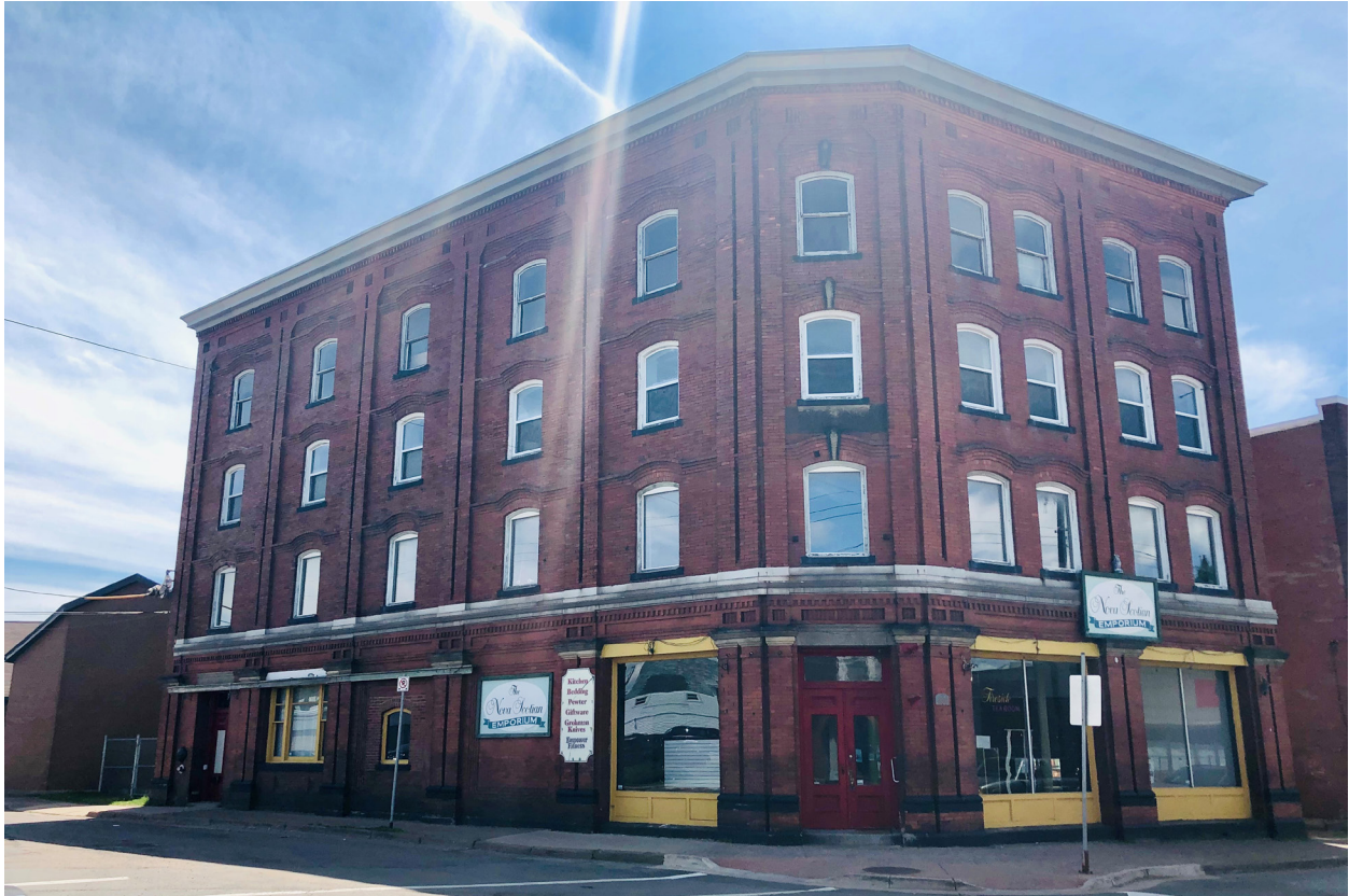
880 Prince Street looking southwest from Prince Street
