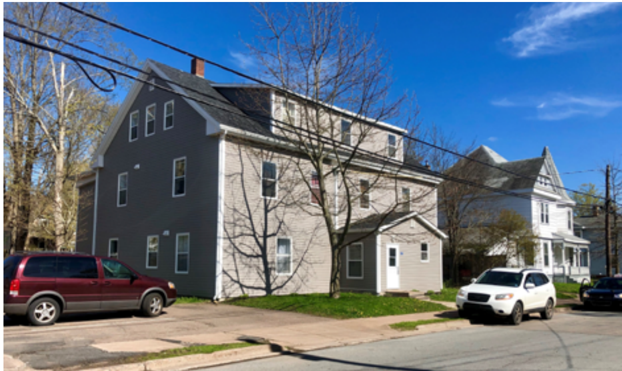
View of the subject property looking southeast from Dominion Street
