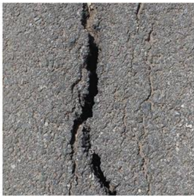
Linear crack
